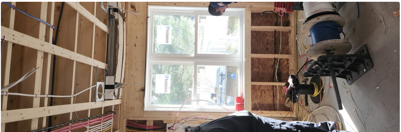
A real Bluestone jobsite — structured wiring rough-in on an active project.
